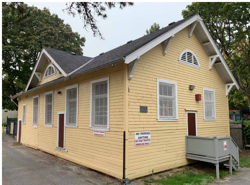
Side/rear; Henry Hudson wooden school building (1912)
