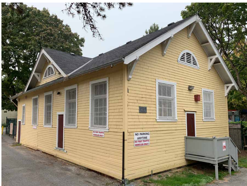
Side/rear; Henry Hudson wooden school building (1912), originally a Manual Training School
