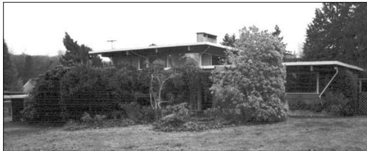
Narod house, north elevation
