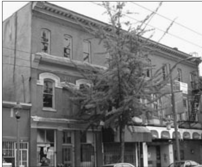
The Wing Sang looking east: Because of its narrow stairwells, furniture was winched through the second-storey door beneath the date stone.
