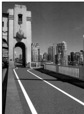
Deck level (note aluminum railings)
