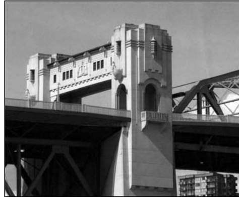
Outriggers with 'Pinch Point' at towers
