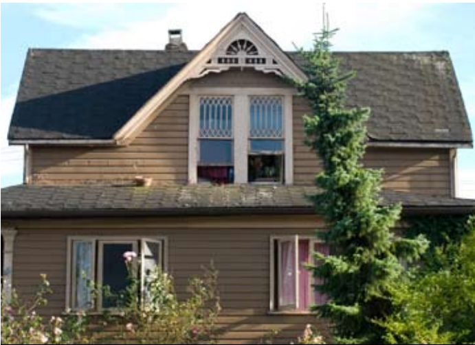
House (1905) at 304 West 5th (Mount Pleasant); on the block for demolition to make room for a BC Hydro substation.
