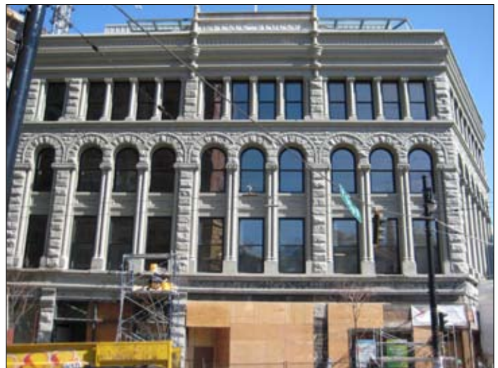
2008; Almost complete with full facade restoration (replication of missing ornamentation, etc.)
