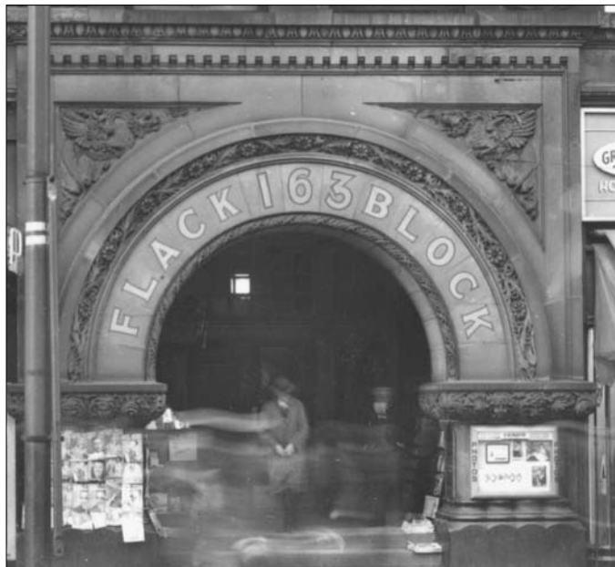
One of the few photos showing the original entry arch in detail. This image served as the basis in recreating the replica archway in stone.
