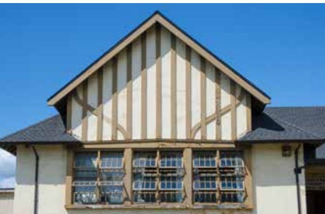
Simon Fraser Elementary School Annex (1929)
